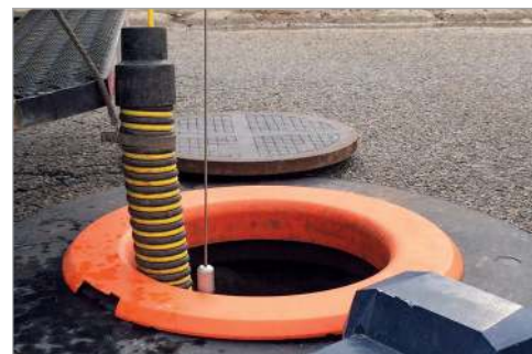
Sewer jet hose and camera protection
