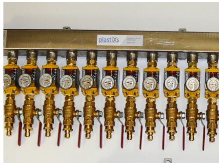
Wall Mounted Return Manifold Assembly with Mechanical Flowmeters and Brass Ball Valves for Laser Cooling Application
